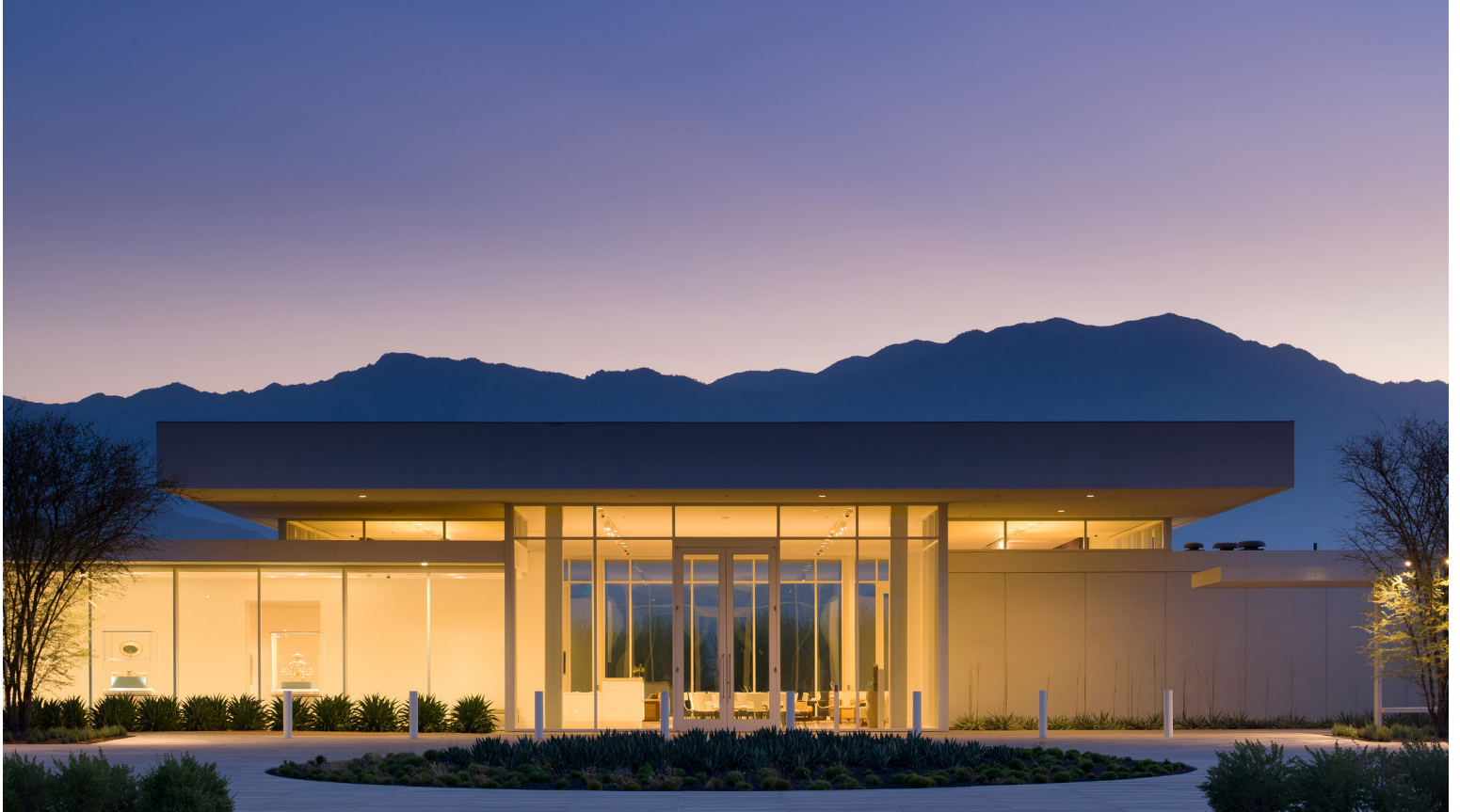
The Interpretive Center blends a modern aesthetic with the rich beauty of the Sonoran desert surroundings.
