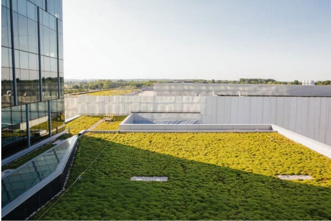
A green roof at the Air Products headquarters. Credit...Michelle Gustafson for The New York Times
